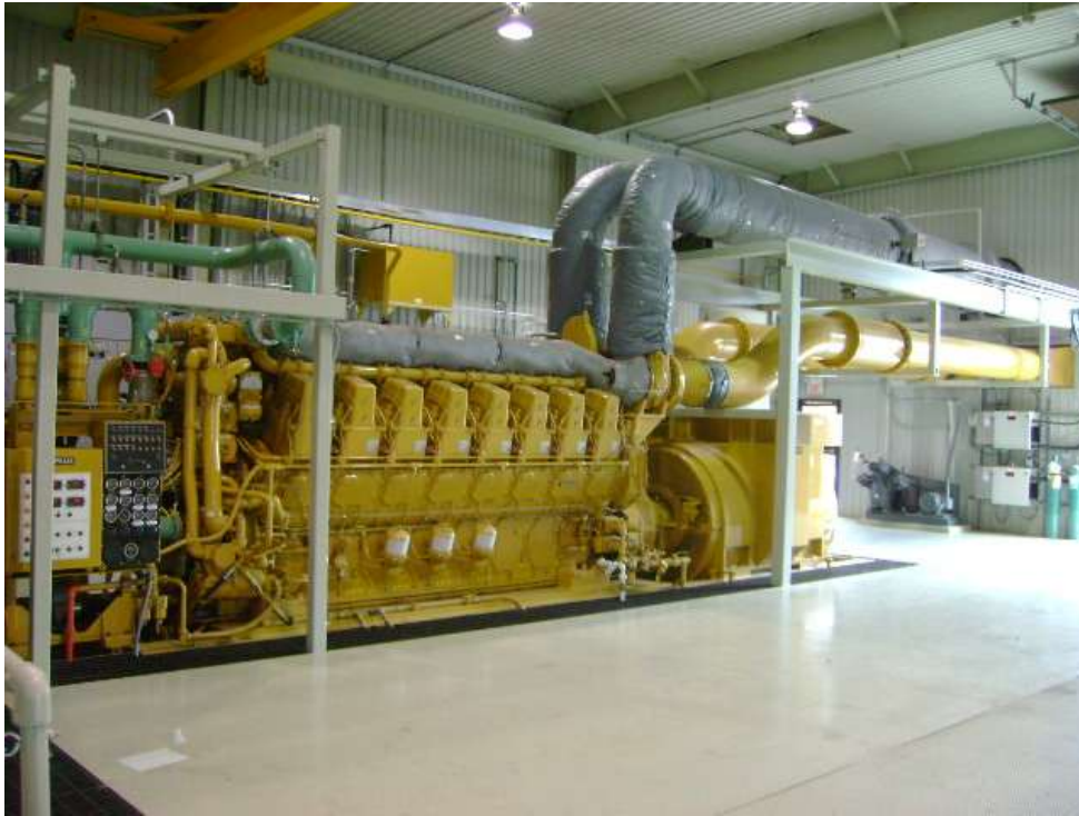
View from Inside
